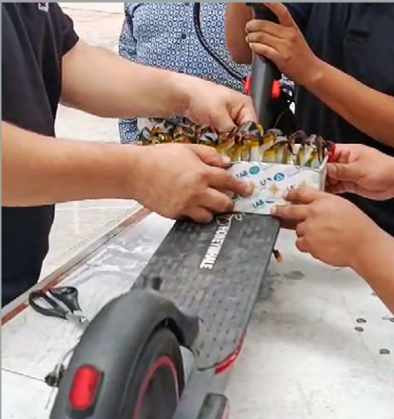
Installation of lithium batteries in scooters
